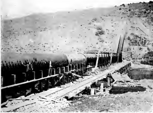
FIG. 6.—WOODEN STAVE PIPE AND BRIDGE.
